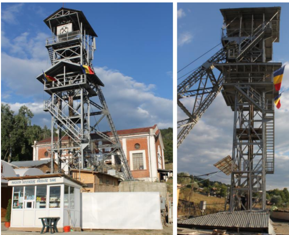
Figure 3. The extraction installation tower from Unirea shaft
