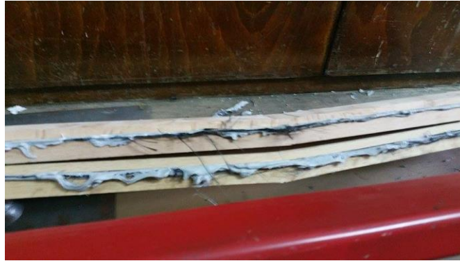
Fig. 3. Reinforcement application: two sheets of carbon fiber
