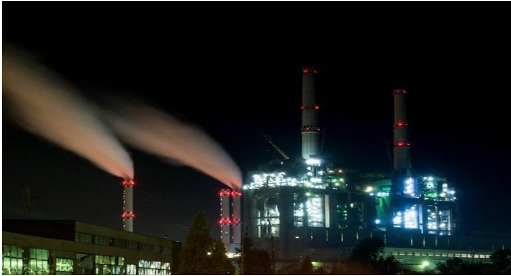
Fig. 1. Rovinari thermoelectric power plant
