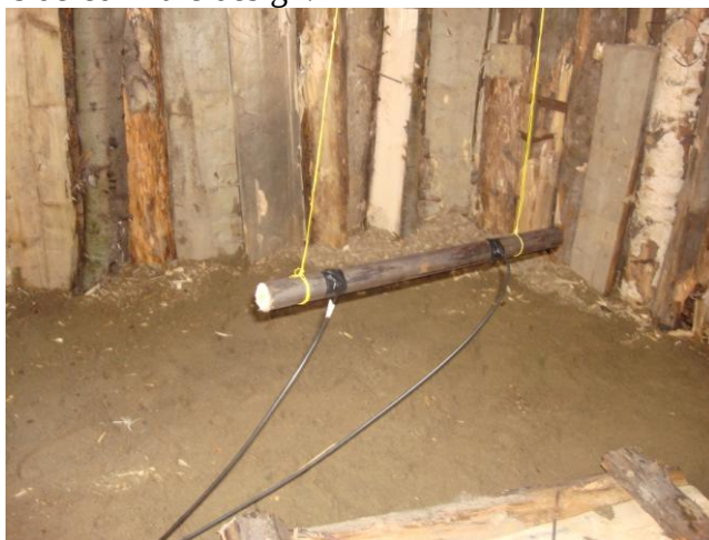
Figure 3. Confined explosive charge placed in bunker – ready to blasting
