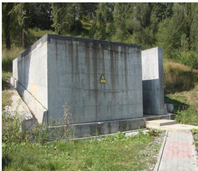
Figure 1. General view of the blasting facility (bunker)
