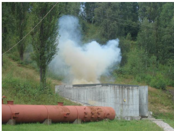
Figure 2. Fumes resulted after a blasting operation in the bunker
