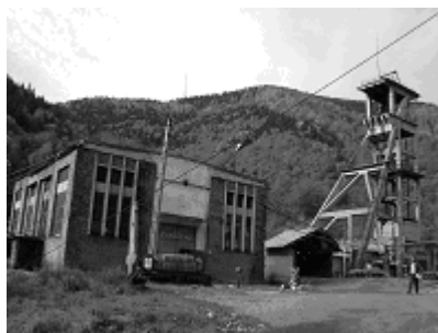
Fig. 2. Extracting installation „Auxiliary well no. 2“
