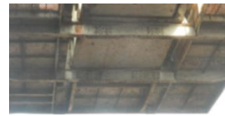
Support beams and cabin floor
