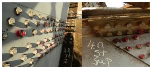
Fig.5. Bookmarks with the red paint of the screws that vibrates.
