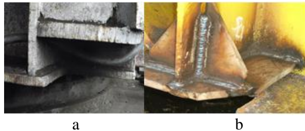
Fig.3. Execution of lifting bracket welding.
