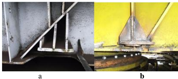
Fig.2. Placement of supports: a-incorrect; b-correct.
