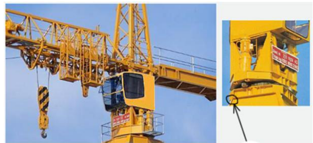
Figure 1. Welding connection between tower and slewing ring of tower crane
