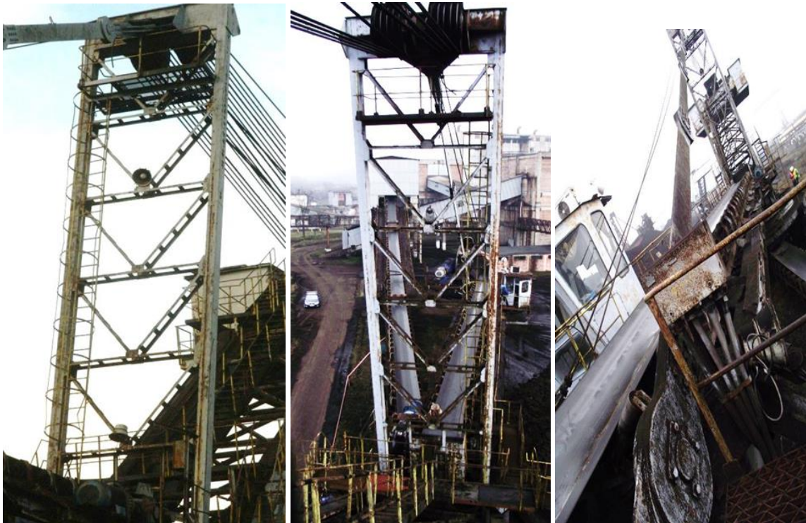
Front view from below
