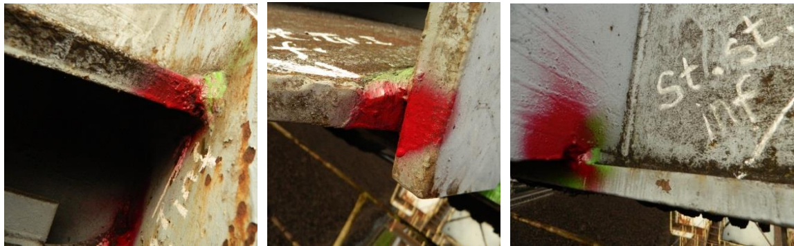
Fig.4 Incomplete welds
