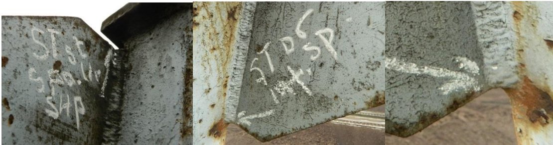
Fig.6 Pendulum executed welds with a size above what is required
