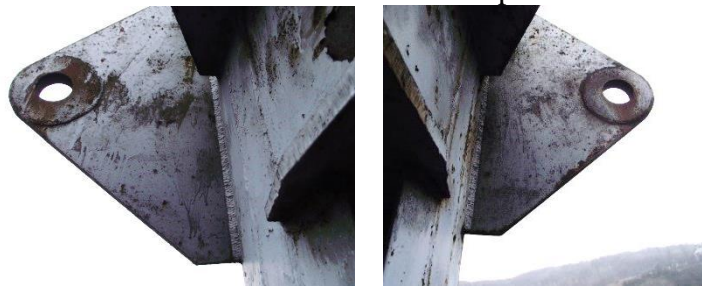
Fig.7 View of the eyelet of the cable change lever
