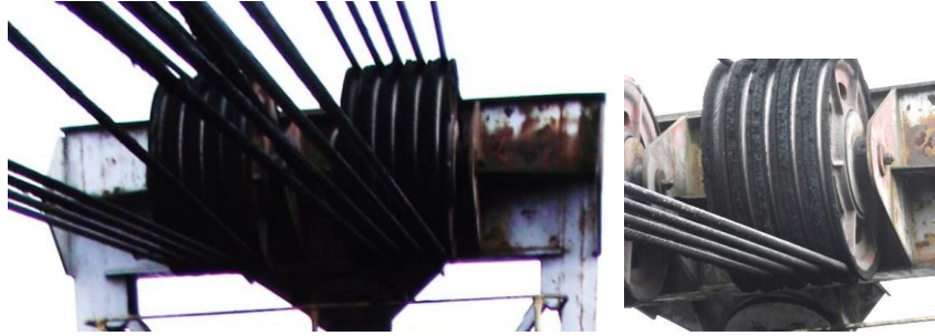
Fig.1 Rust attacked the paint
