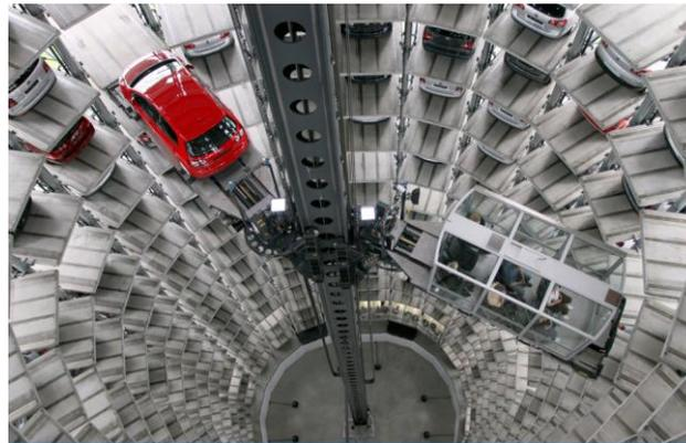
Fig.1 The elevator with a robotic actuation used for the execution of parking lots with high capacity
