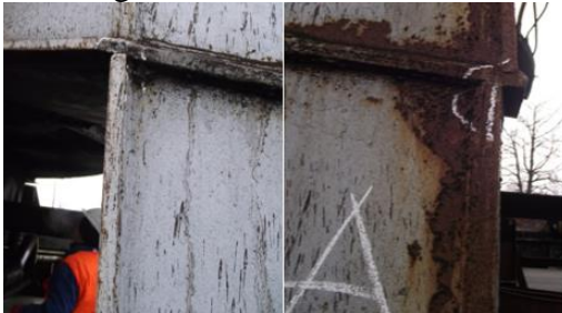
Fig. 5. Tripod support on the rolling mechanism „A”
