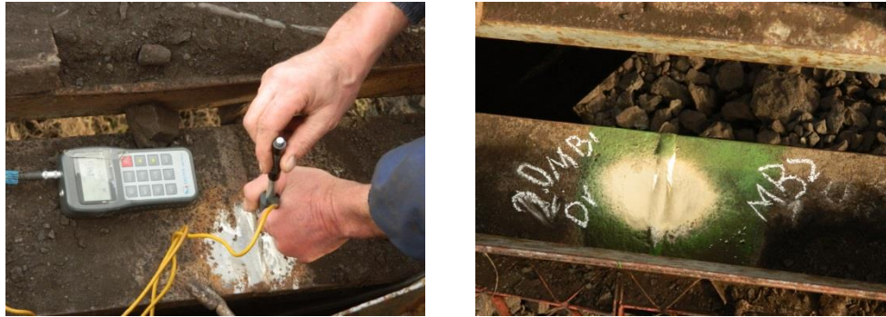
Fig.4 P33-P34 welded joints
