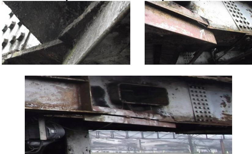
Fig.5. Lateral diagonals from "Section I" with unadjusted parts at lower sole grip
