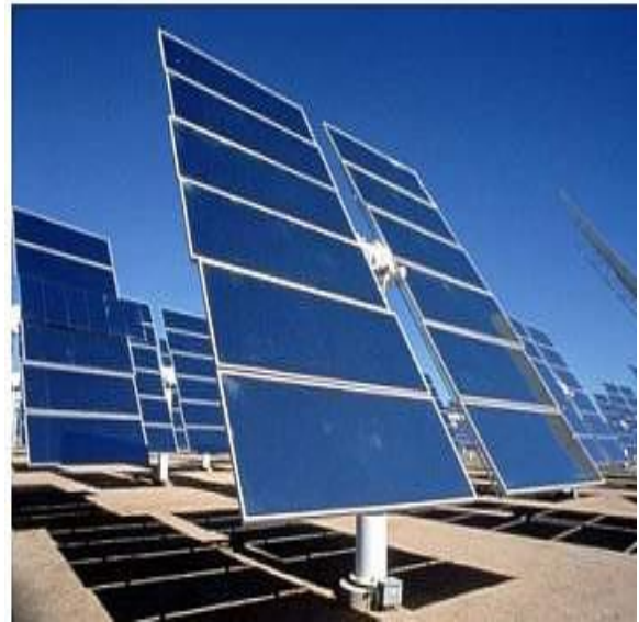
Figure 3. photovoltaic park in tracking system with 2 axis
