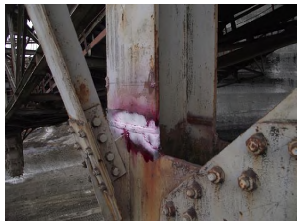
Figure 4 - Application of the developer to the micro-cracked area
