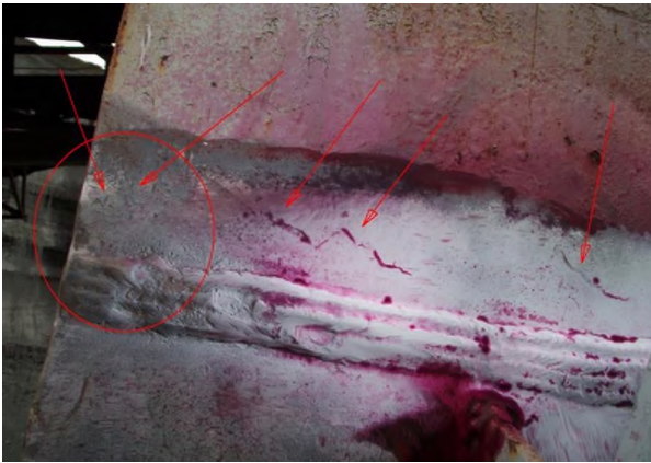
Figure 5 - Microcracks in the area of ZIT and fatigue
