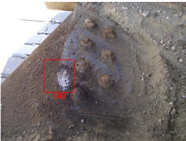
Figure 11 a. Cleaning the area for ultrasonic control
