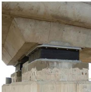
Fig. 3 Seismic isolators LASTO-LRB
