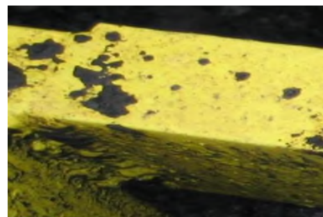
Figure 8. Non-conformity - diagonal in the lower field
