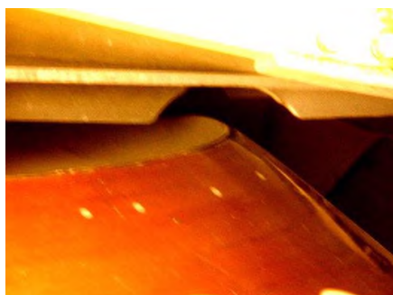
Fig.10. Non-conformities - the soleplate of the upper area.
