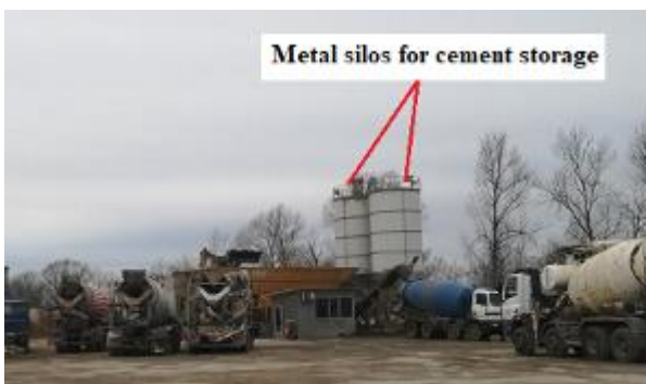
Fig. 2. Metal silos for cement storage
