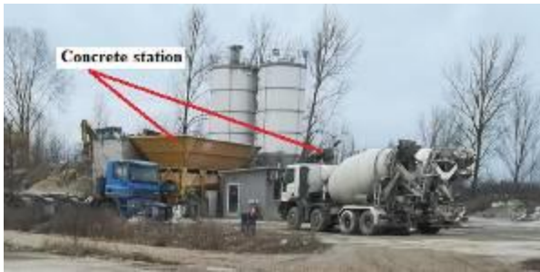
Fig. 1. Concrete and mortar preparation station
