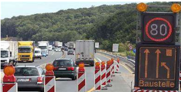
Figure 2. Roadworks on the motorway [23]
