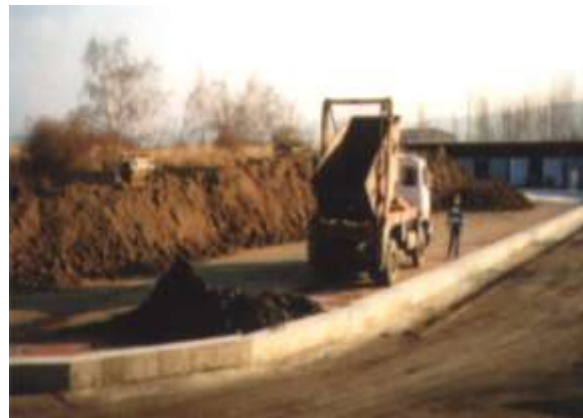
Fig.5. Submission soil impermeable platform
