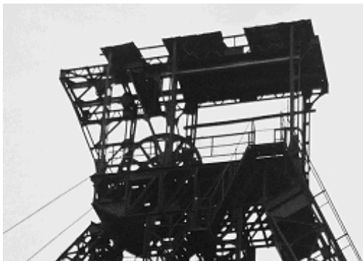
Figure 3. Extracting pulleys
