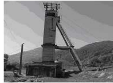
Figure 3. Installation tower „Auxiliary well Jieț“
