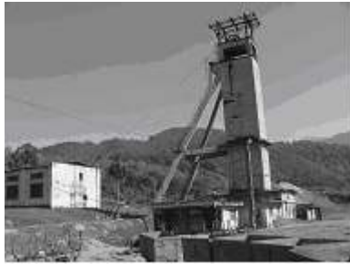
Figure 1. Extracting installation „Auxiliary well Jieț“
