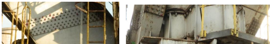
Fig.4 Gripping the rotating platform side and back
