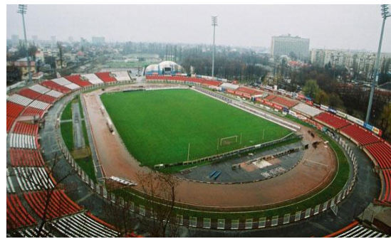
Fig. 9. Amenajarea unui stadion Fig. 9. Construction of a stadium
