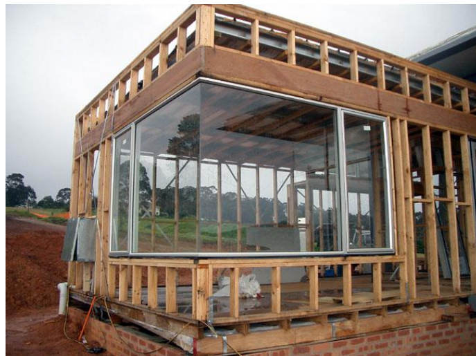
Fig. 1. Typical corner window during construction
