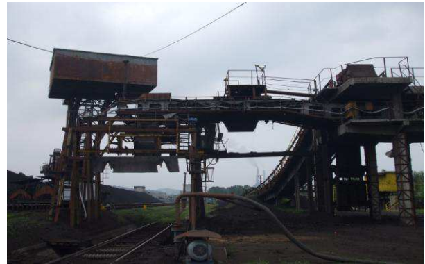
Fig.no.3 Loading point.
