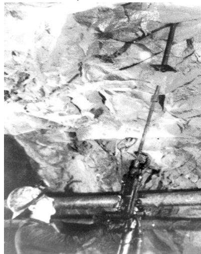
Figure 4 Manual drilling installation fitted with a perforator which can be easily fixed on a telescopic column
