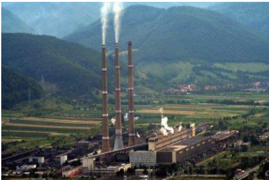
Fig.1 Mintia Thermal Power Plant
